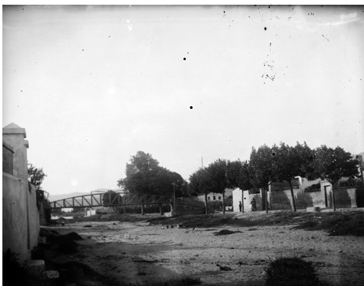
General view of the iron bridge, ca. 1910. Author: Emili Martínez i Passapera. Collection: Martínez - Planas. SAMLM - Municipal Archive Service of Lloret de Mar. S.T.: 303.023.018.
